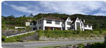
Gap Rest House
